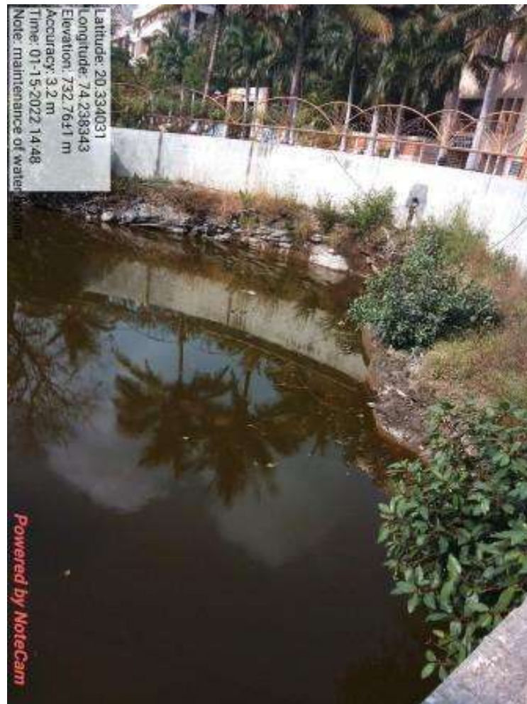
Figure 4. Open well Recharge
